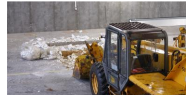
Excavation for new pad foundations
