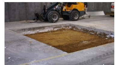
Ready for new concrete
